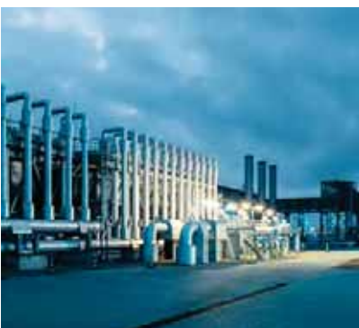
Example of hydrogen plant
